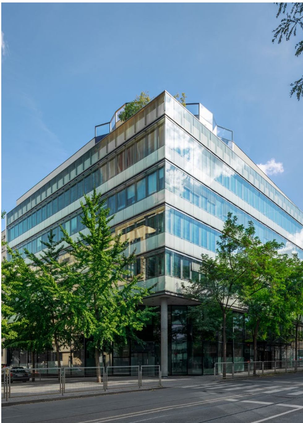
Idea office building – Smíchov
